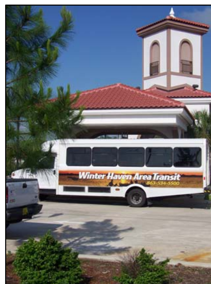
Winter Haven's downtown terminal is an example of a transit hub.
